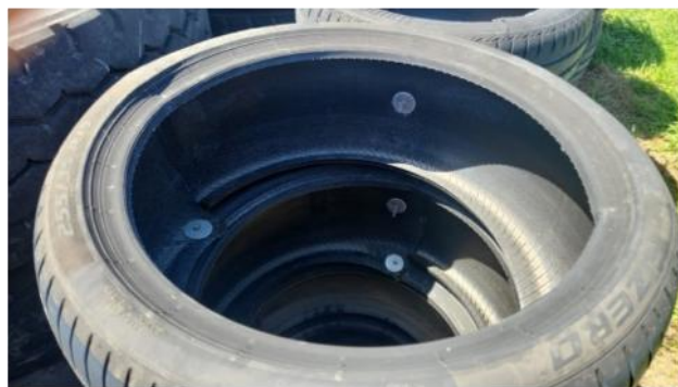
TEK Screws with washers being used to build tyre walls.
