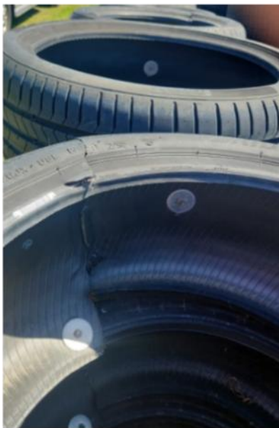
TEK Screws with washers being used to build tyre walls.
