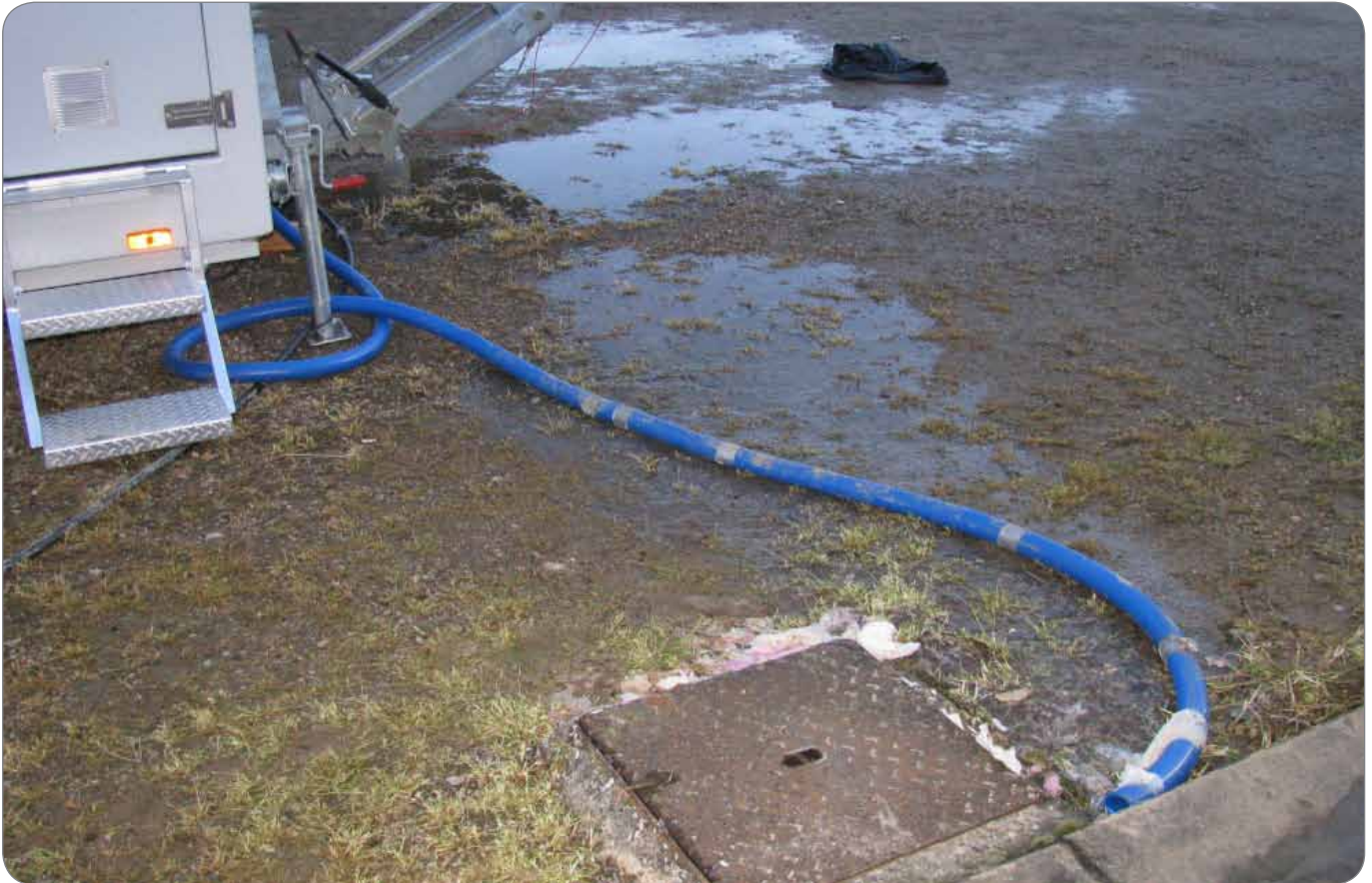
Above: Inappropriate disposal of waste water causes pollution and unhygienic conditions.
